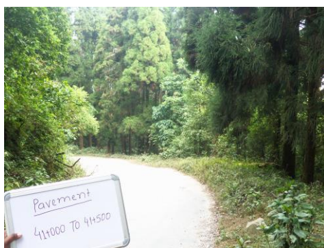
Pavement At km 41+500
