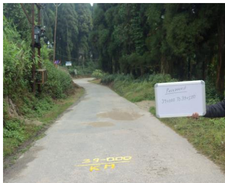
Pavement At km 39+000
