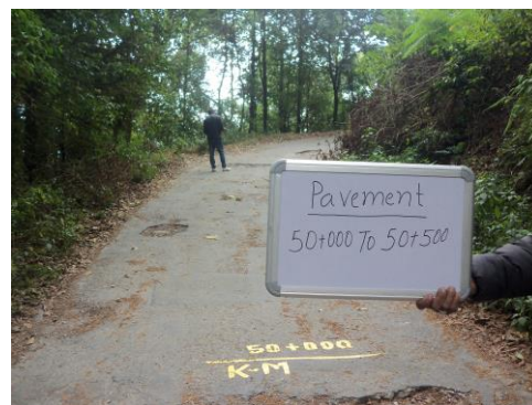
Pavement At km 50+500
