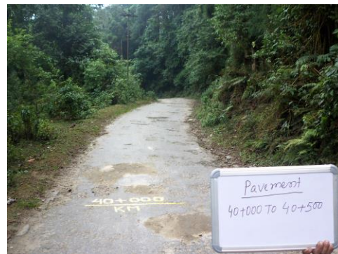
Pavement At km 40+500
